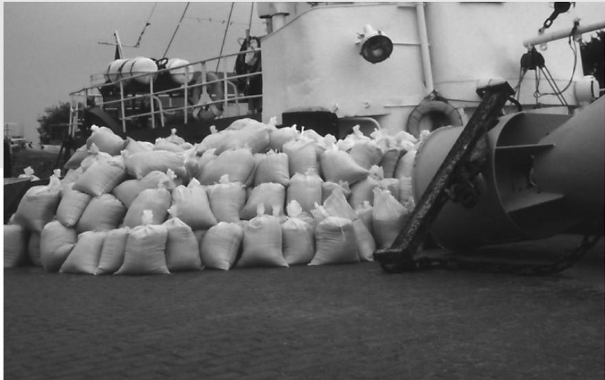
Loads of sandbags were used on the Darsser Cog site to level out big height differences prior to the protection with the polypropylene nets (Thomas Förster).
