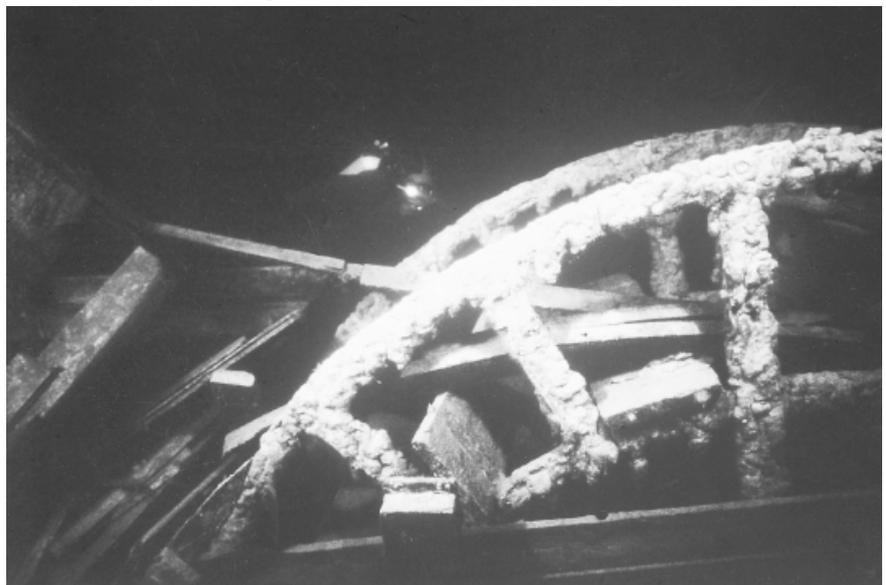
One of the paddle wheels of the E. Nordevall photographed not long after the localization of the ship in 1980. To the left can be seen pieces of the dilapidated wheelhouse (Tony Holm).
