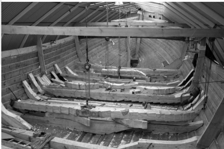
By building a full scale replica of the “Poeler Cog” in Wismar harbour (Germany), late medieval shipbuilding can be visualised (Photo: Roland Obst, Erfurt).
