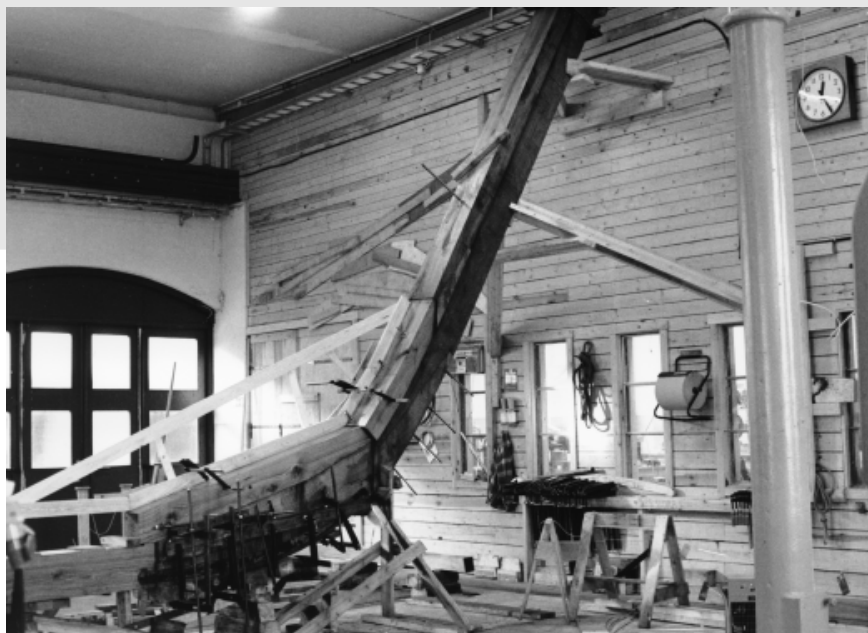
The bow section and the stem post under construction (Photo: Carl Olof Cederlund).
