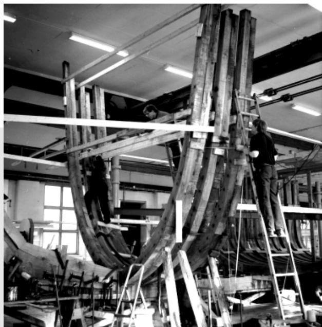
The raising of frames on the keel in the fore section of the hull (Photo: Carl Olof Cederlund).
